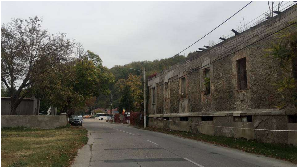
Fig. 7 Aspects of existing vegetation around the MFS building site
